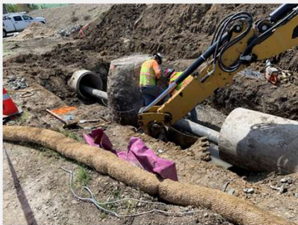
Camp Stoneman Interceptor Repair
