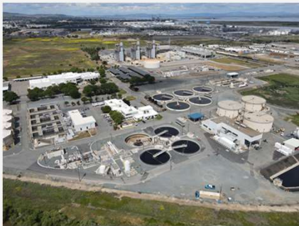
District's Wastewater Treatment Plant
