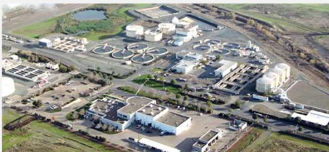
District’s Wastewater Resource Recovery Facility, includes:
