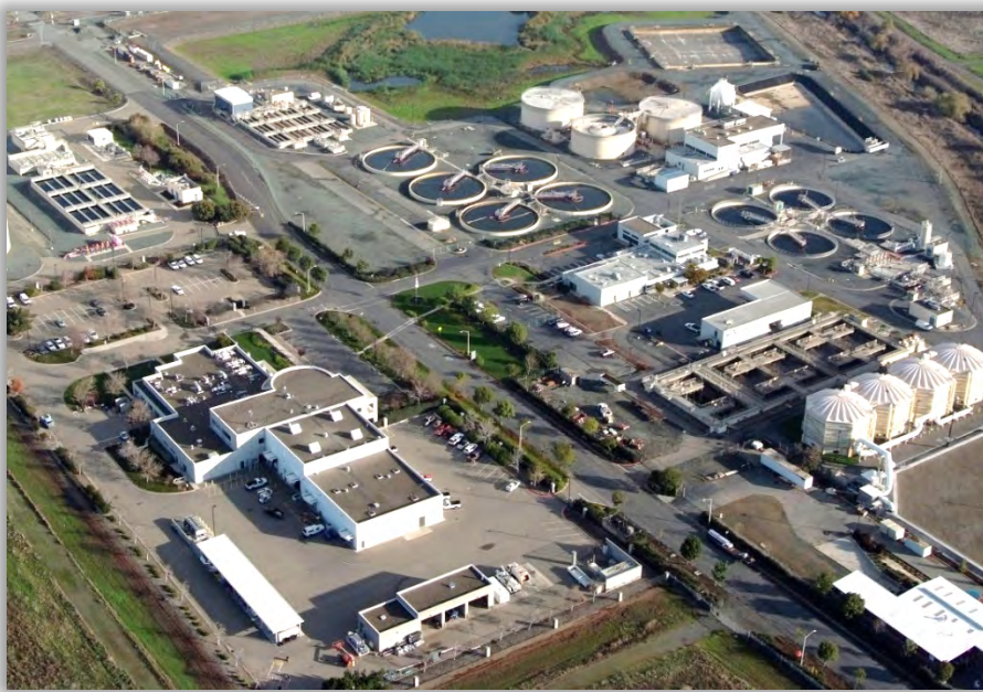
TREATMENT PLANT AND DISTRICT OFFICES
