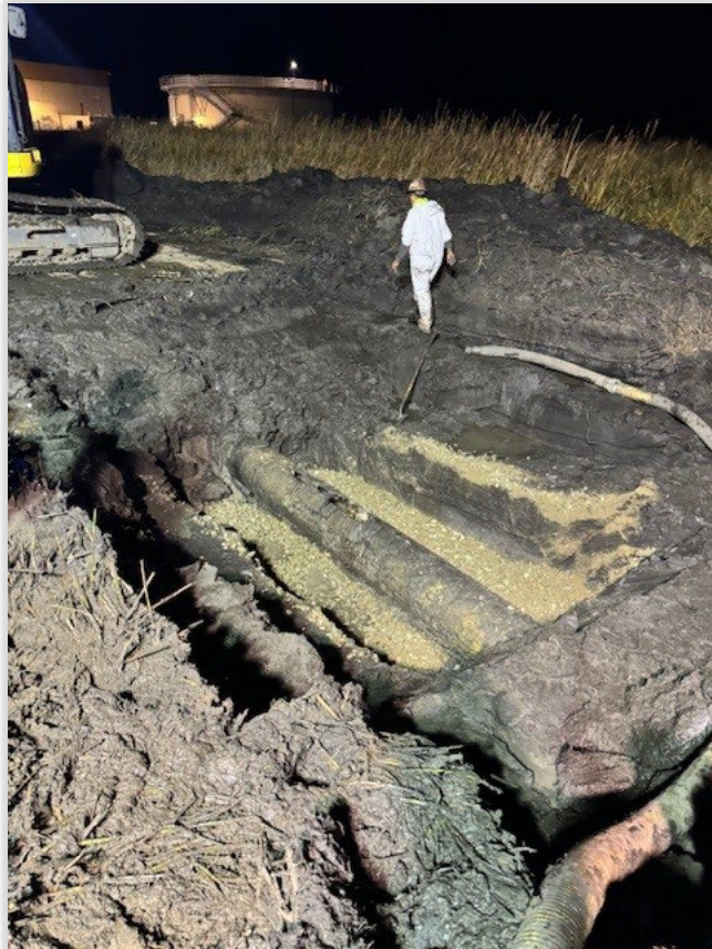
Excavation Work to Expose SAPS Forcemain Failure Point (Tue, 12/3)
