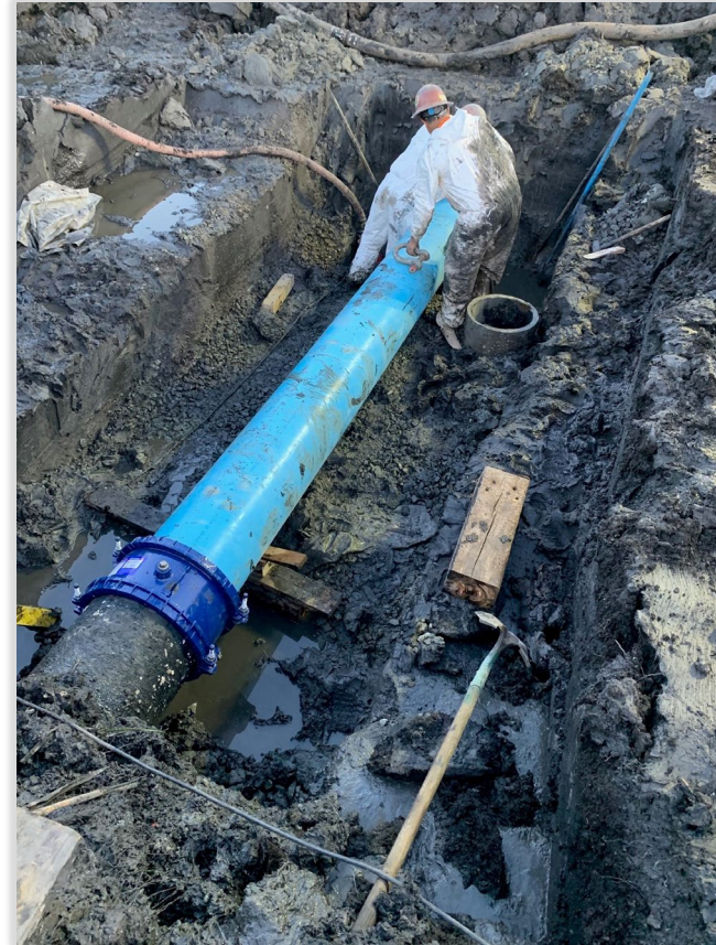
Installation of 20-ft PVC Section to Repair Forcemain (Wed, 12/4)
