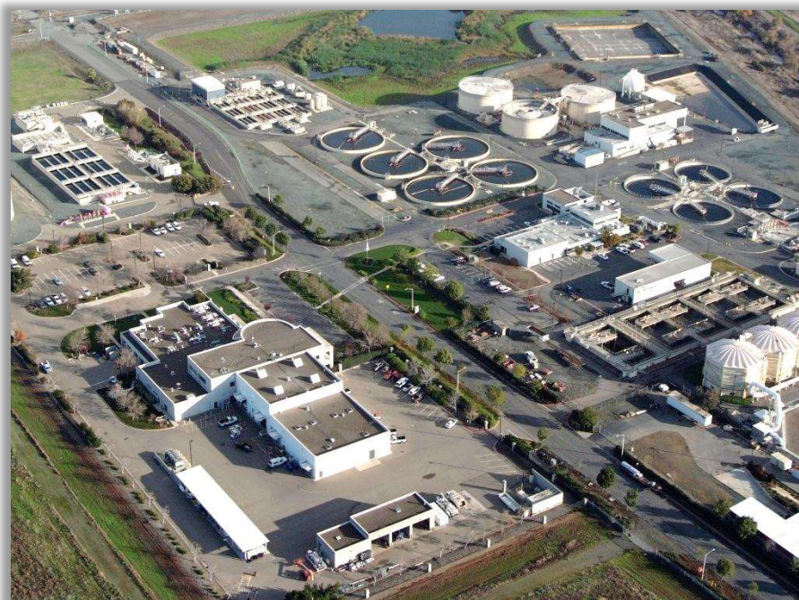
Treatment Plant and District Offices
